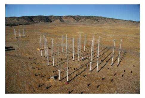
Dabiri's smaller vertical-axis turbines can be clustered very close together — like a school of fish — and each turbine's power coefficient doesn't drop much when placed in close proximity. In fact, the vertical-axis wind turbines can feed off of one another, resulting in increased efficiency in some cases.
